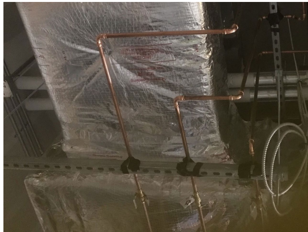
Food Court Renovation
