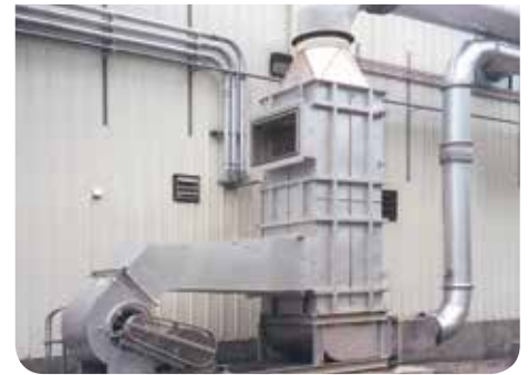
Thermo-Z® heat exchanger indirectly cools gas from two production lines before entering a baghouse.
