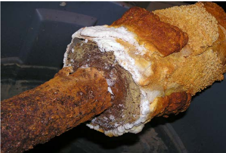
Pipe & insulation after 2 years
