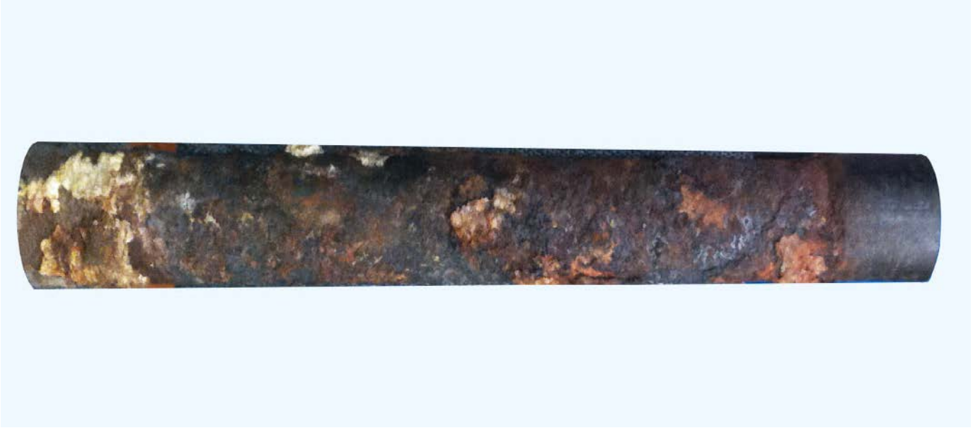
Pipe with Grease Tape after 10 Years
