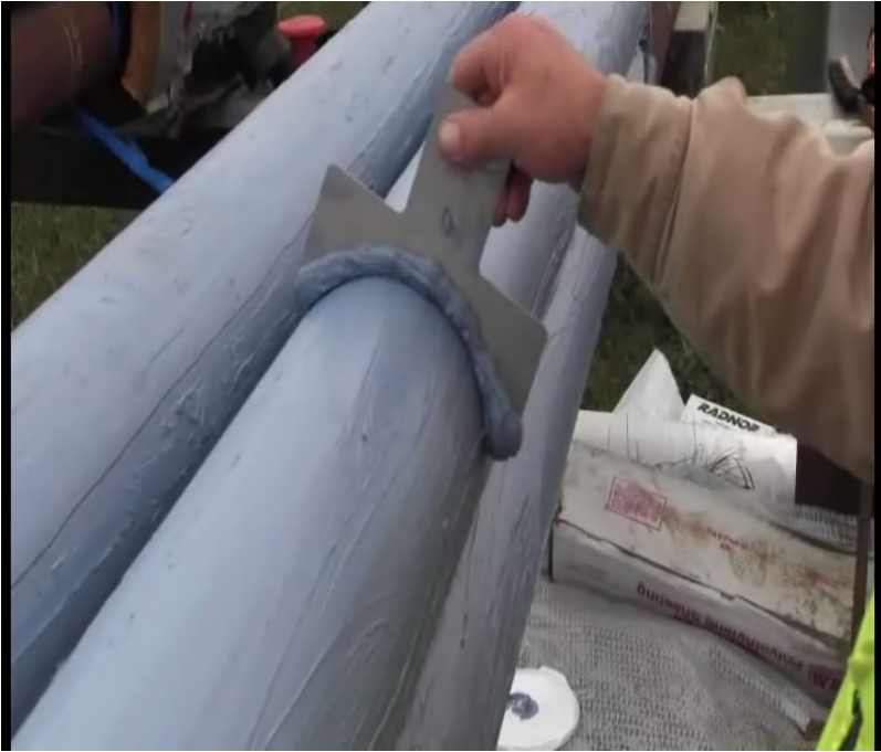
Picture 3- Using Calibrated Trowel to Apply Gel
