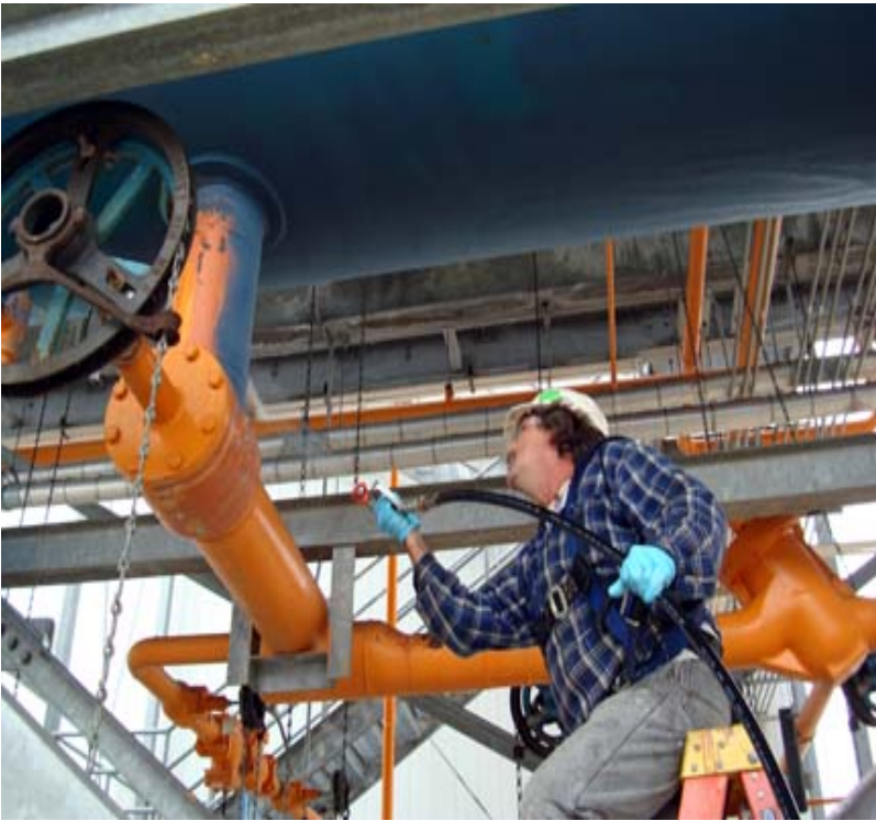
Picture 4- Gel Being Spray Applied
