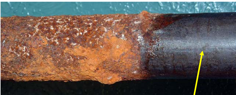
2 year test pipe after Reactive Gel is cleaned off
